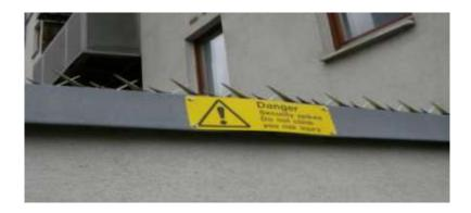
*Figure 1: Spikes atop a barrier wall act as a deterrent to people trying to climb over the wall*<sup>3</sup>
