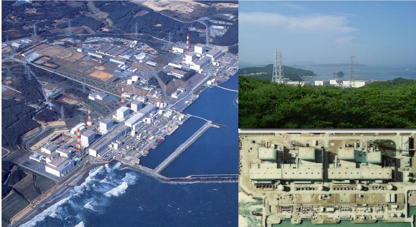
The plant before the accident on 11 th Mar 2011
