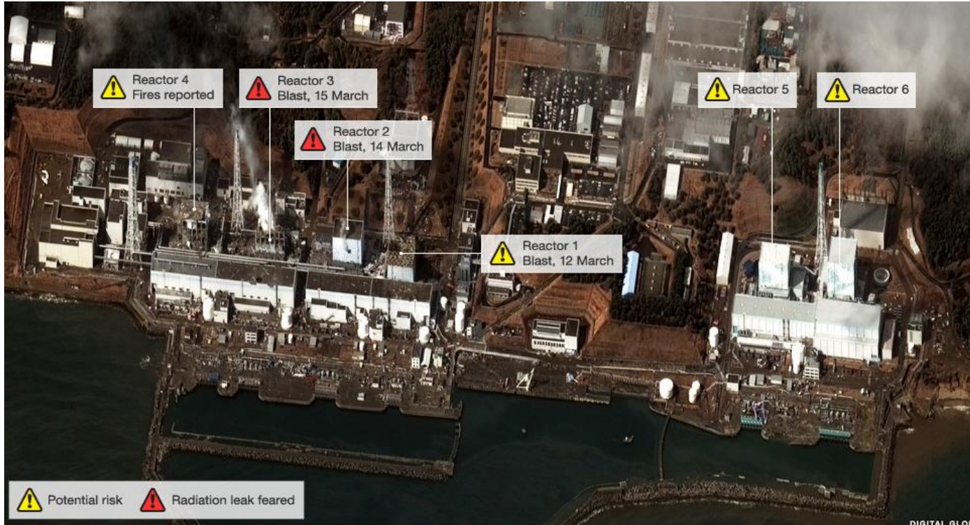
Daiichi NPP after multiple hydrogen explosions (16.03.2011)
