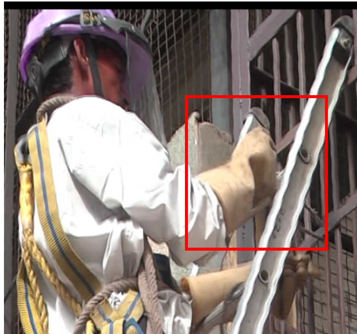
Tying the ladder with rope
