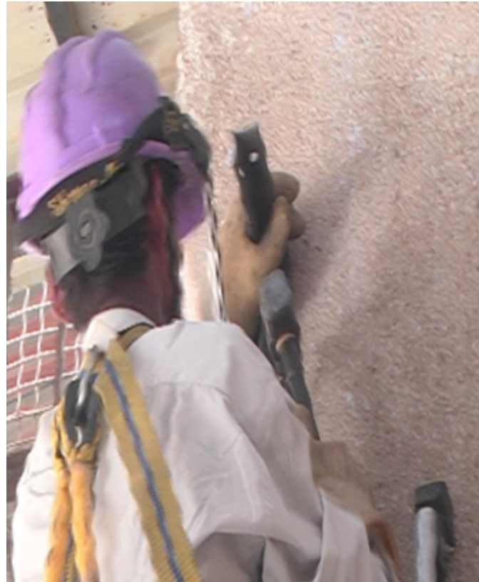
Piercing the fasteners of angle bracket with hammer
