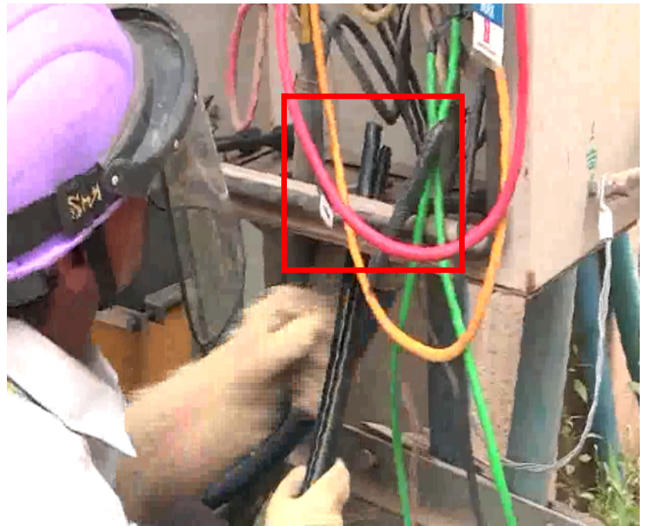
Inserting the cable ends in bus chambers of MCCB
