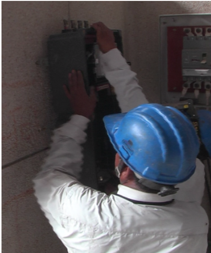
Mounting of meter box
