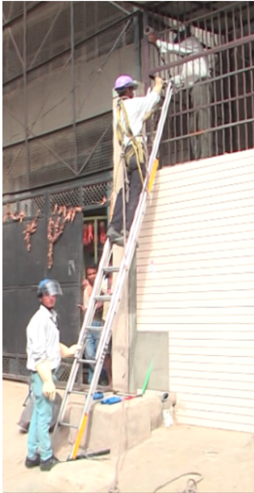
The ladder is set up
