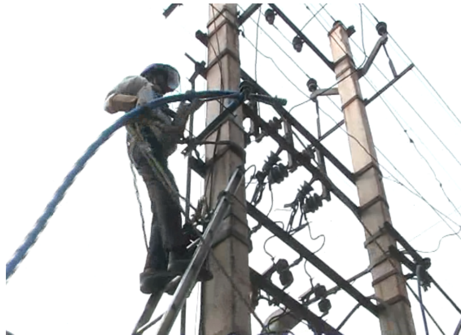
Cable drawing process at Double Pole (DP) structure
