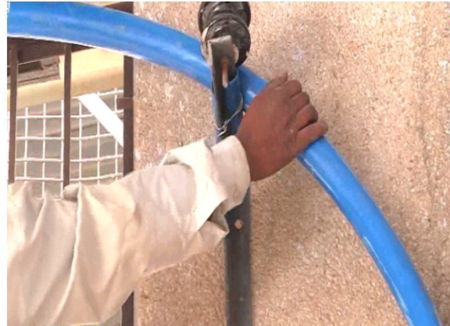
Cable drawing from outside the fence
