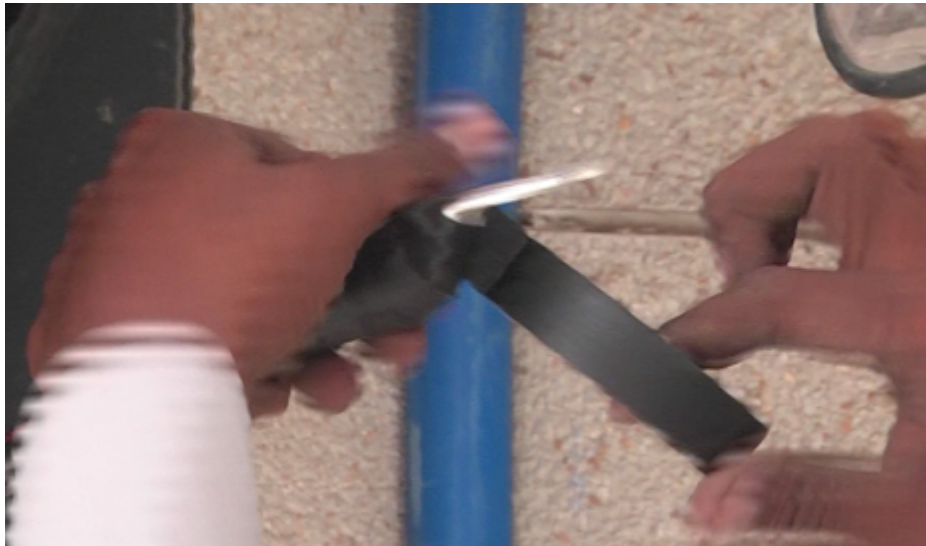
Thimble is covered with insulation tape
