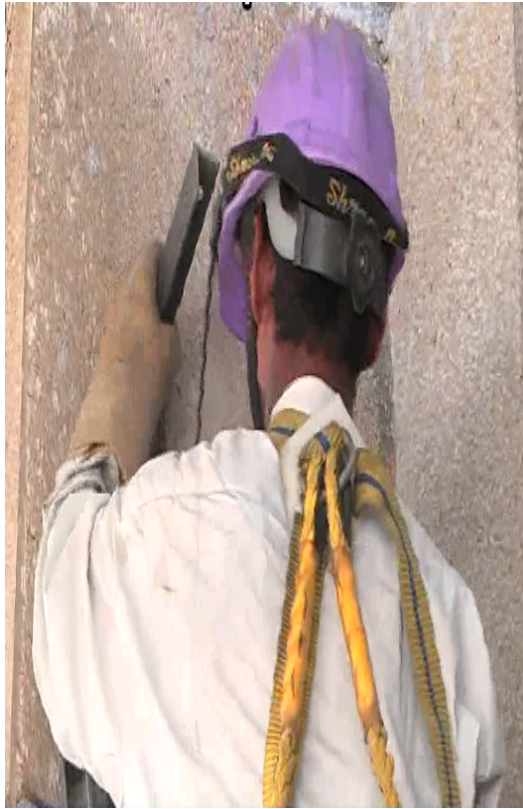
Fixing the angle bracket
