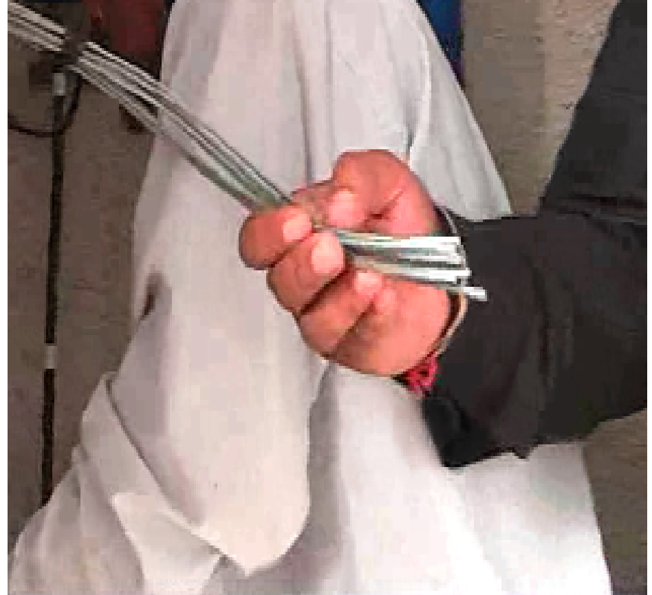
GI wires of the armouring of cable
