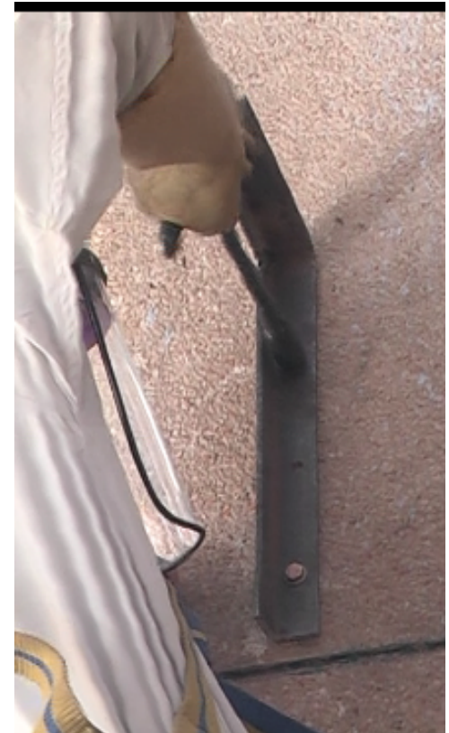
Tightening the bolts with box spanner
