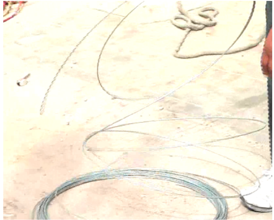
The GI wire is used as catenaries to guard the cable
