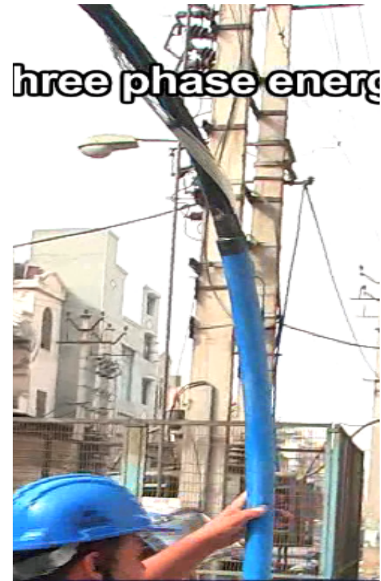
Cable with the PVC pipe
