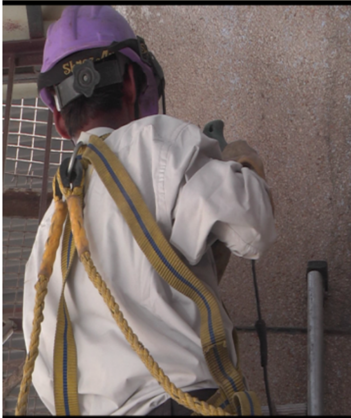
Drilling to fix the angle bracket
