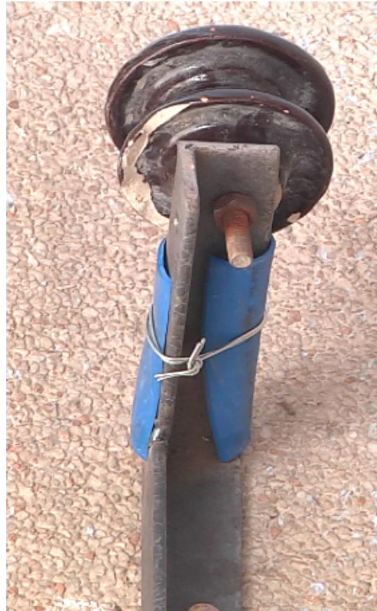
Fixation of shackle insulator on angle bracket
