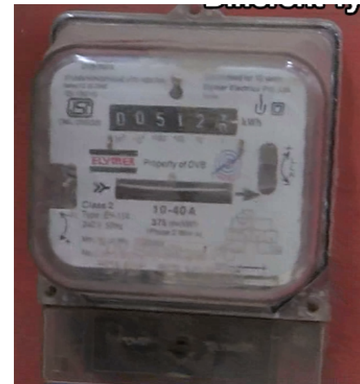
Electromechanical meter with polycarbonate body
