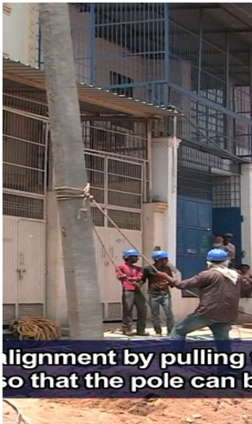
Vertically lifted pole over the pit
