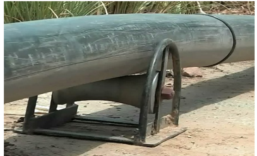
Cable is loosened easily over the roller stools
