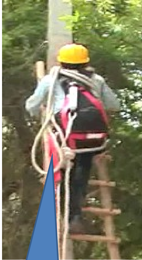
Lineman climbs up the pole with safety PPE and rope
