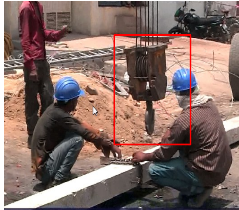
Pole will be balanced vertically when lifted with the help of the hook
