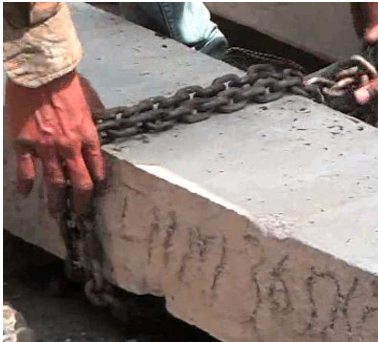
Chain is placed at the centre of the pole
