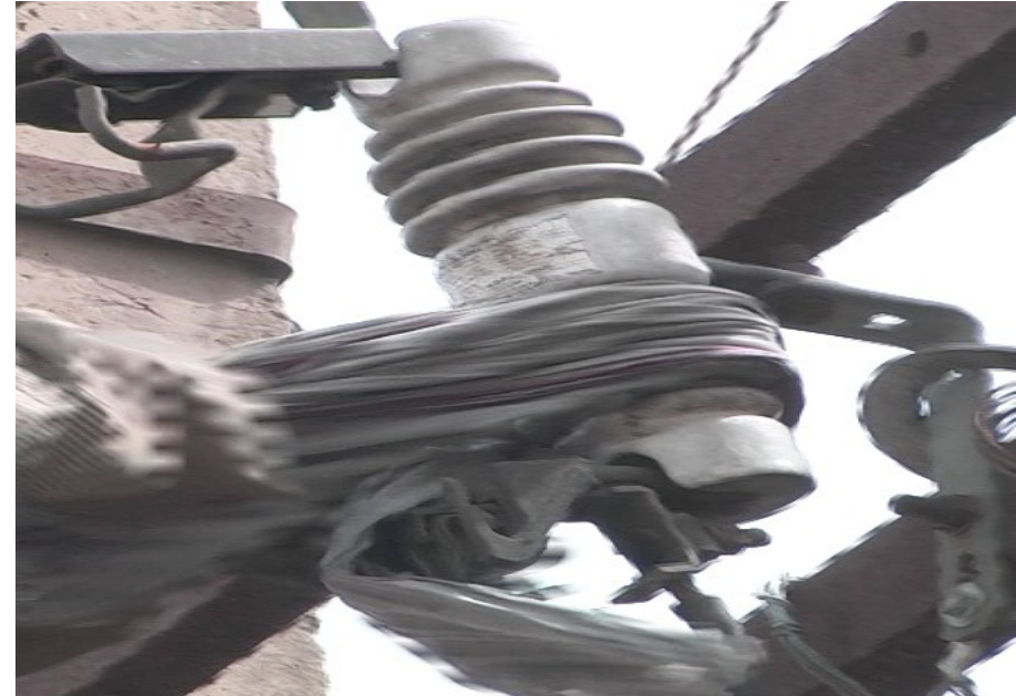
Cleaning HT and LT bushing of transformer
