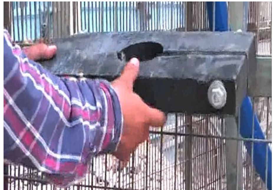
Wooden cleat is fixed to the fencing or MS frame
