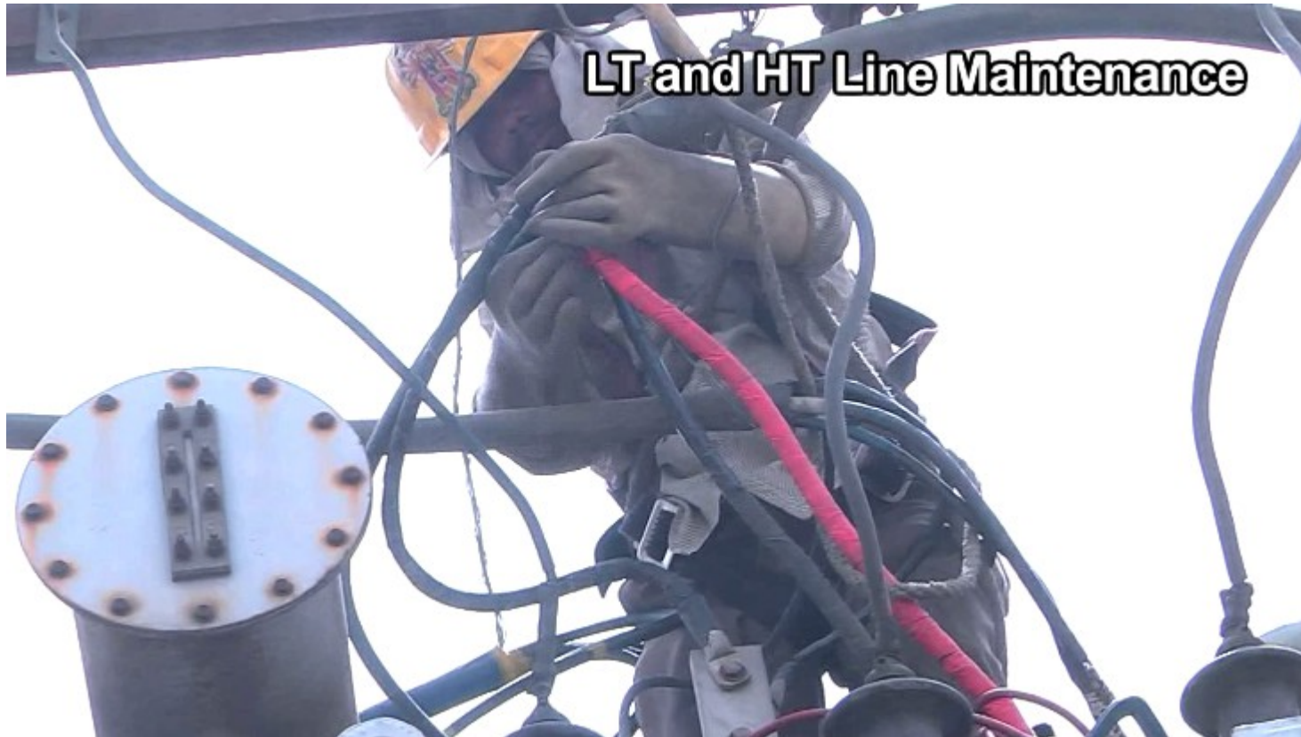
Lineman repairing the LT cable joints
