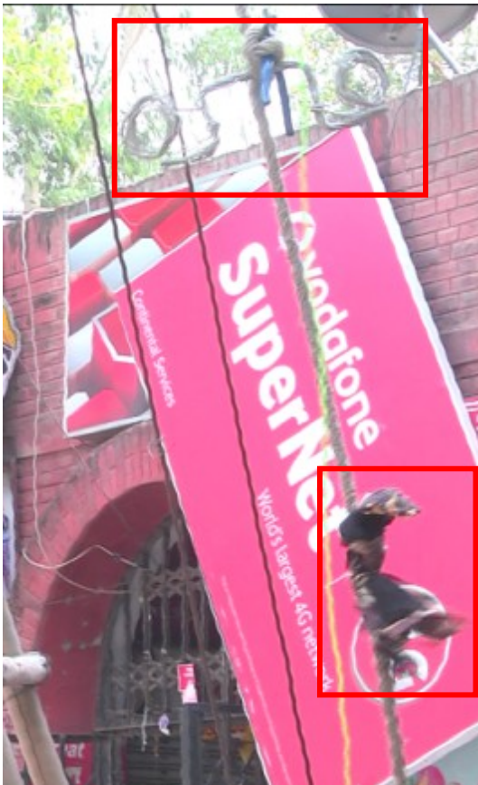
Helper is providing D-clamp and a duster through rope
