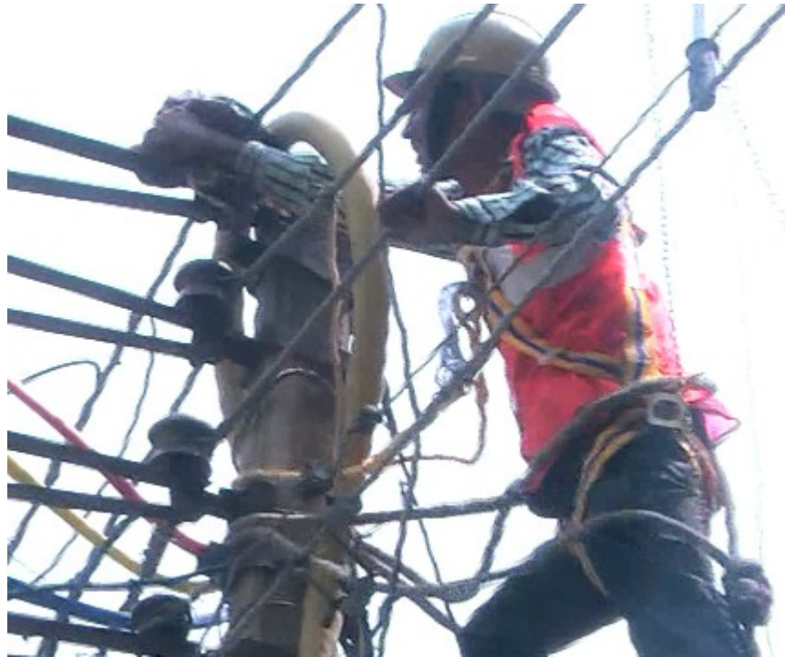
Lineman removing the dust from the insulators
