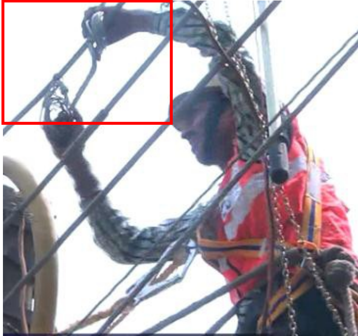
Fixing the D-Clamp
