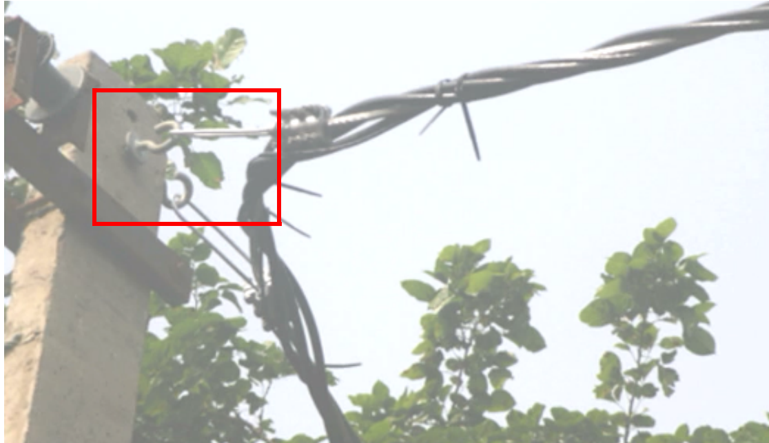
Anchoring Clamp
