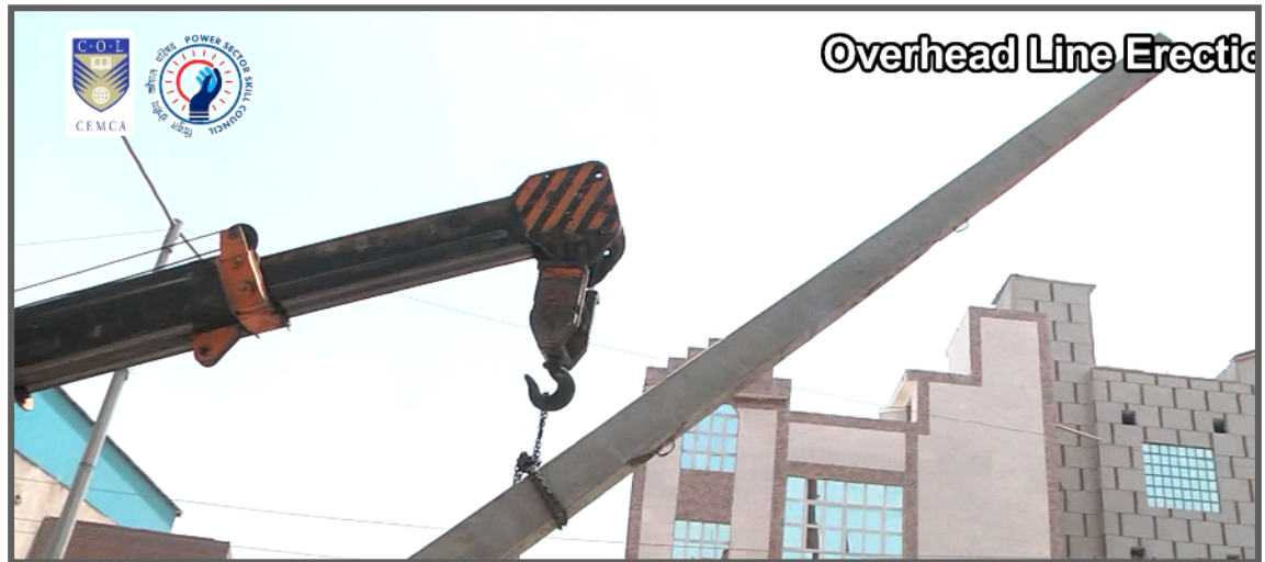
● Pole being lifted using cantilever system
