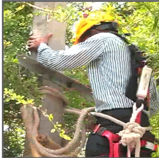
● Tightening the cross arm
