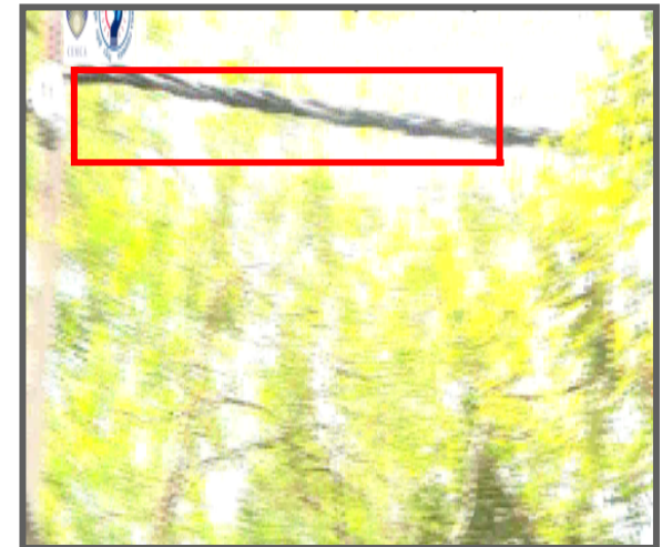
● Cable is pulled over the branches through pulley
