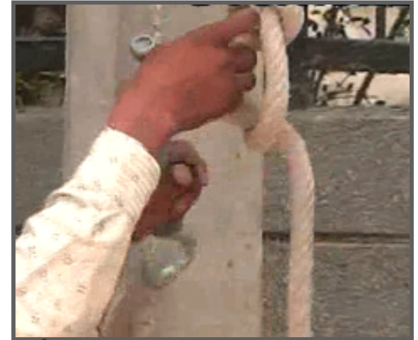
● Sending tools through the rope
