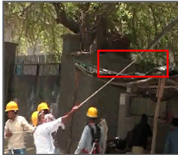
● Ground crew pulling cable with rope
