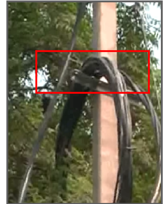
● Cross arm fixed on the pole
