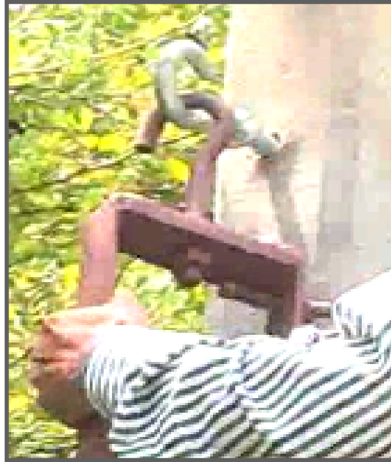
● Placing pulley on eye hook
