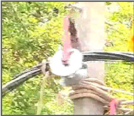
● Inserting cable into the pulley
