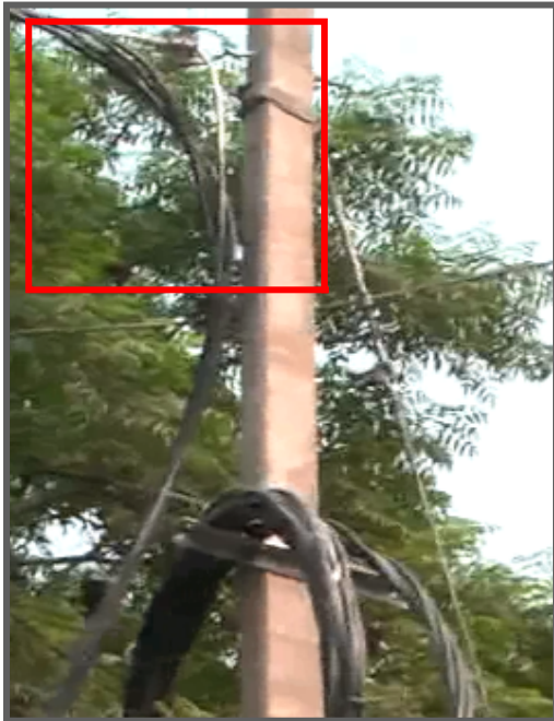
● Stay wire fitted at the end of the pole
