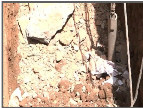
● Pit where the pole has to be erected
