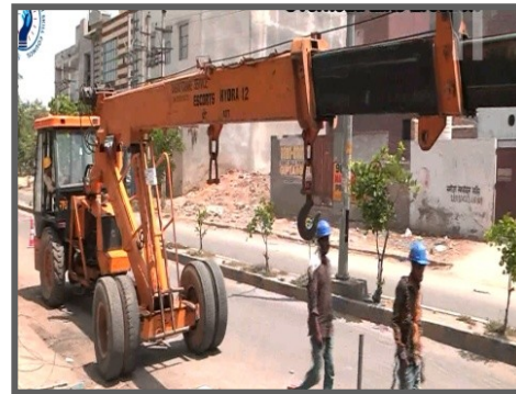
● Crane to lift the pole
