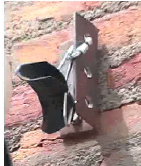
Suspension hook is fixed to the angle bracket
