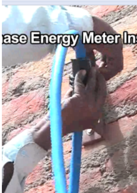
Insertion of cable in the suspension hook
