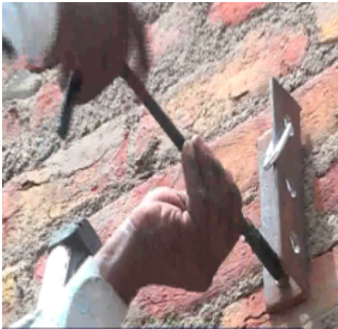
Fixing of angle bracket on the wall
