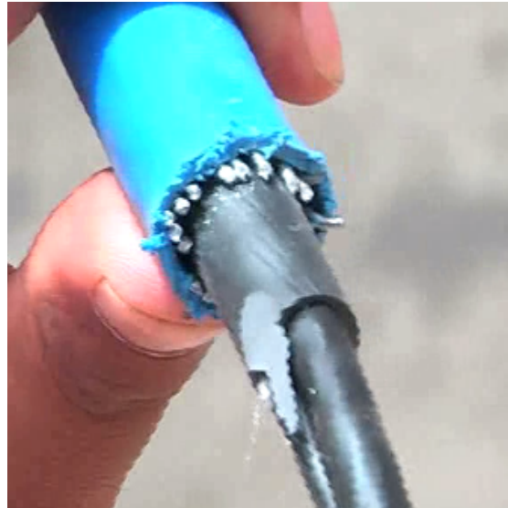
Outer most PVC sheath of service cable is peeled
