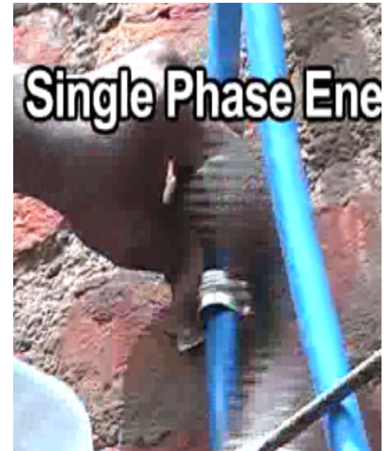
Fixing of saddle
