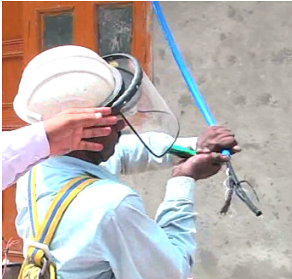
Creating jumpers on the cable
