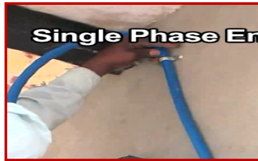
Clamps the cable on wall with saddles
