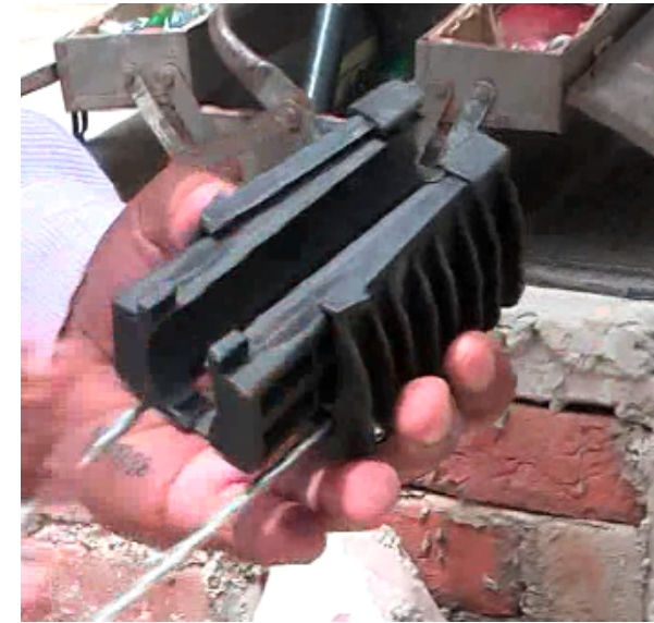
Anchor is pressed to bind and grip the cable
