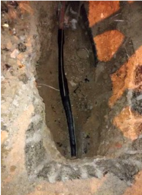
Pit for new cable joint
