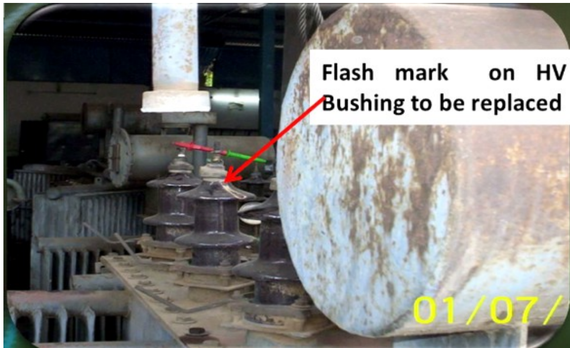
Fault identified on HV bushing
