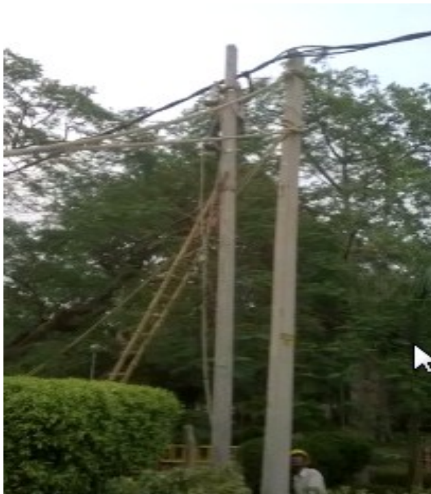
Replacement of uprooted pole
