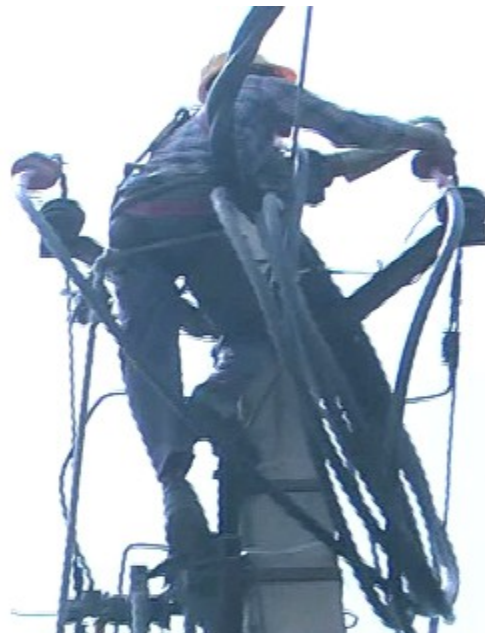
Lineman replacing the burnt cable with the new one
