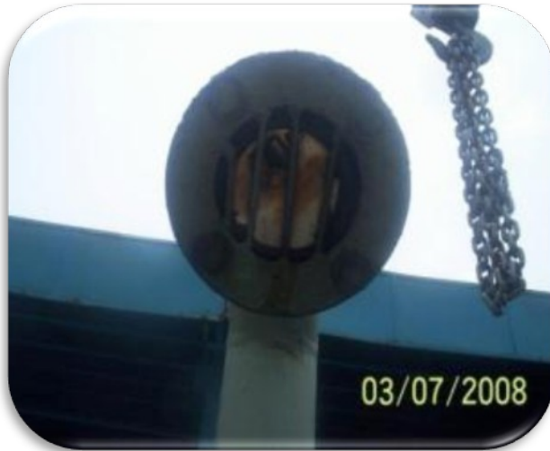
Explosion Vent Diaphragm
