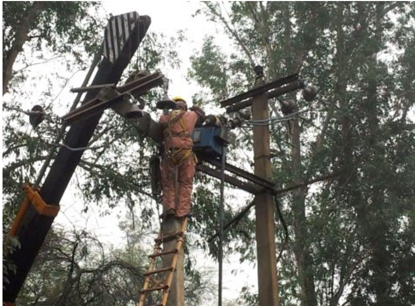
Lineman removing the HT disc insulators
