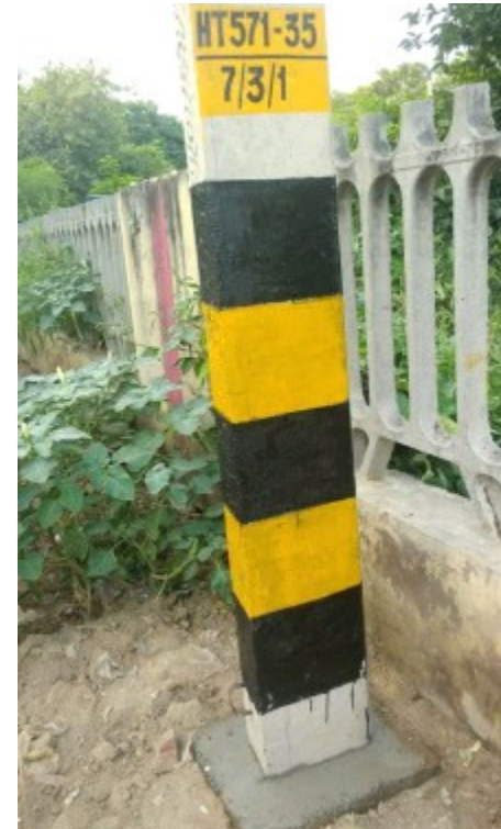
New pole is grounded on cement mortar
