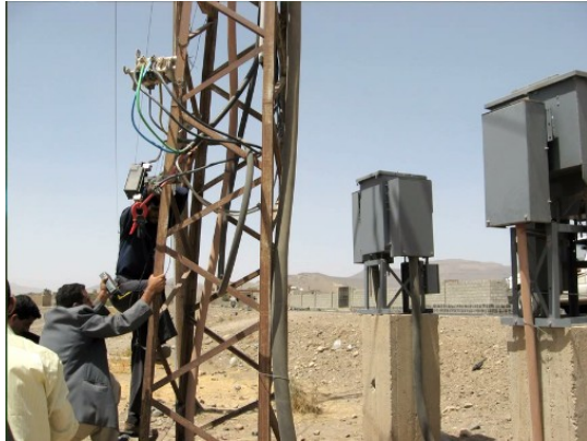
Checking the line condition using multimeter
