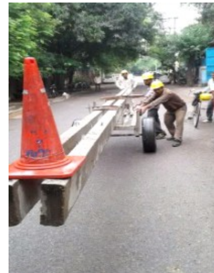
Carrying LT poles on a pole cart
