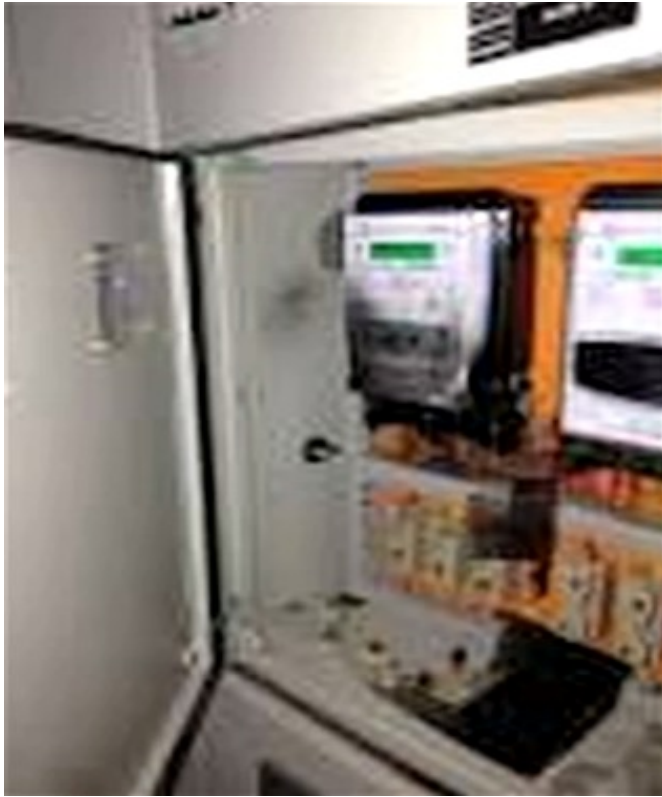
Defective meters, where consumer's supply is affected
