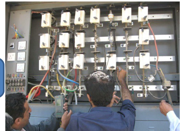
Checking the line condition using multimeter and clamp ON meter
