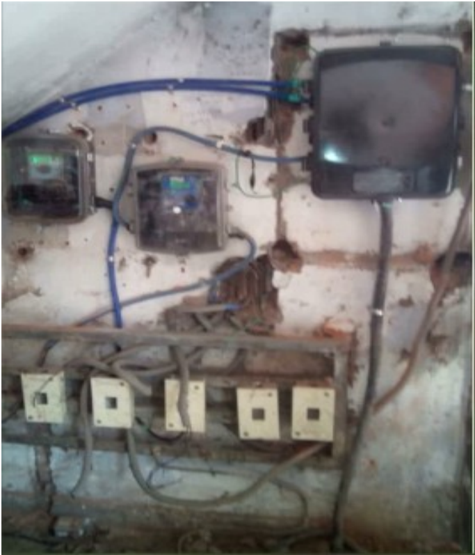
Defective meters, where consumer's supply is affected
