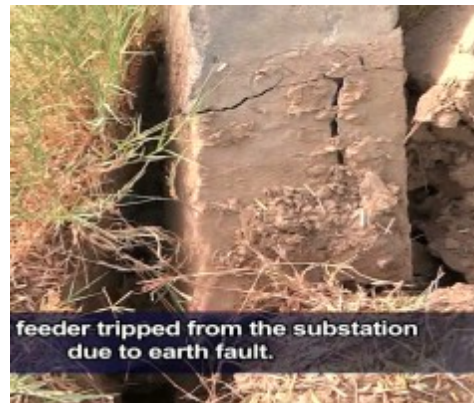
Tripped LT feeder
