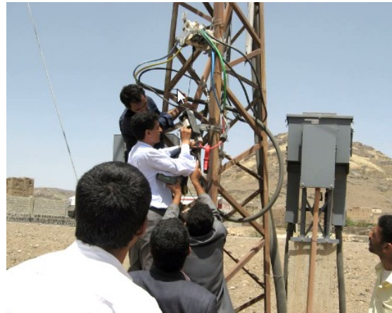
Checking the line condition using multimeter and clamp ON meter
