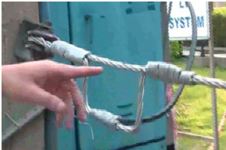
Neutral conductor, the 5th one
