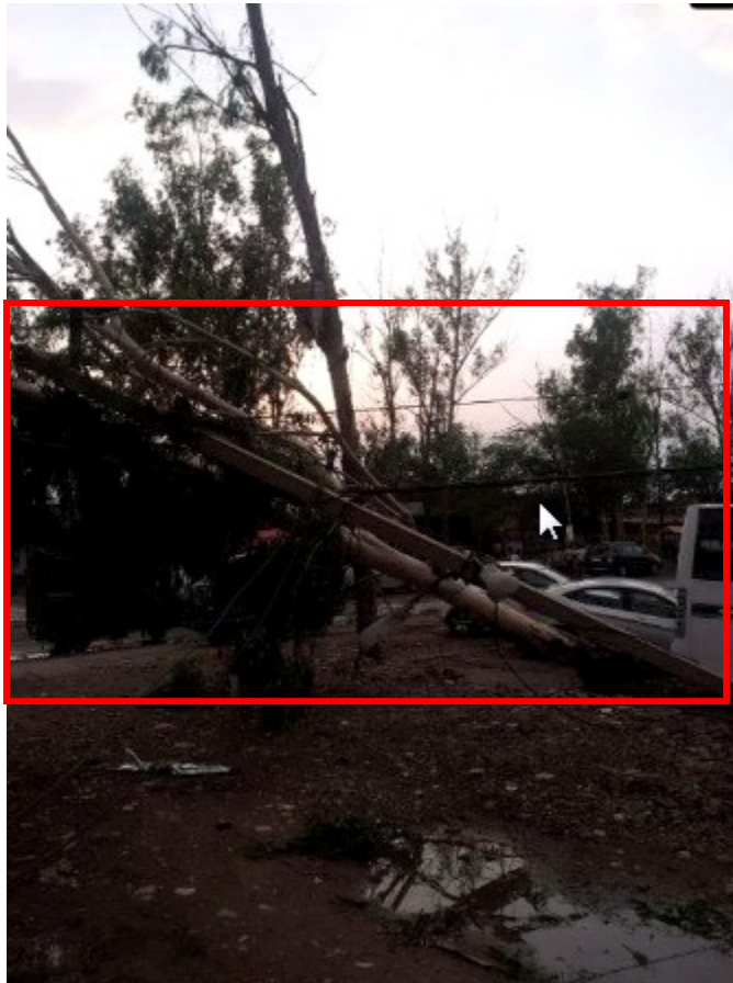
Uprooted LT PCC pole
