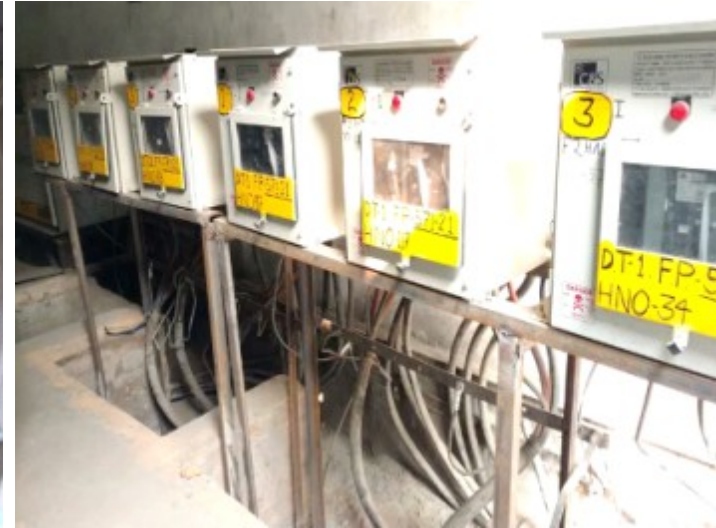
LT panel replaced with new ACB
