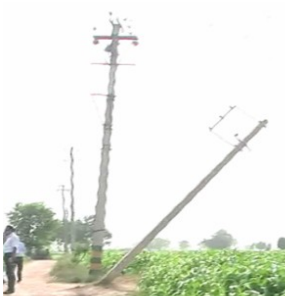
LT PCC pole hit by a tractor
