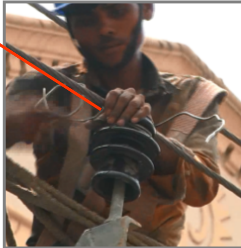
Lineman places the HT wire over pin insulators
