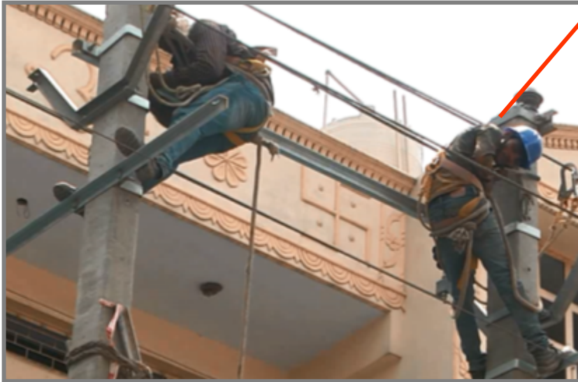
Lineman fixes the aluminium wire over insulator
