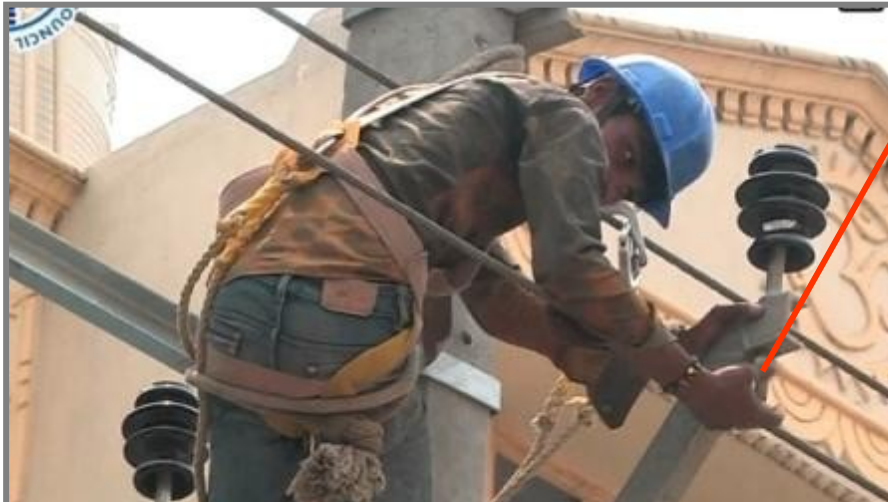
Tightening of Pin Insulator Screw
