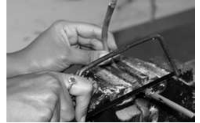
Step 3: Cut the excess length after bending.
