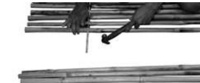
Step 20: Keep adding the bamboo poles to the rod.
