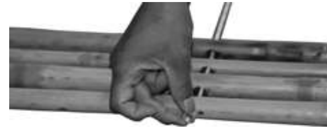
Step 19: Lock with a nut on one end of the rod.
