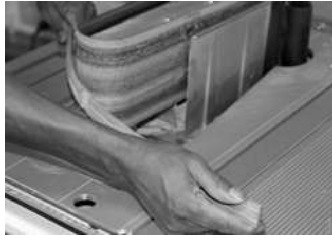
Step 14: Sand it and clean the surface.
