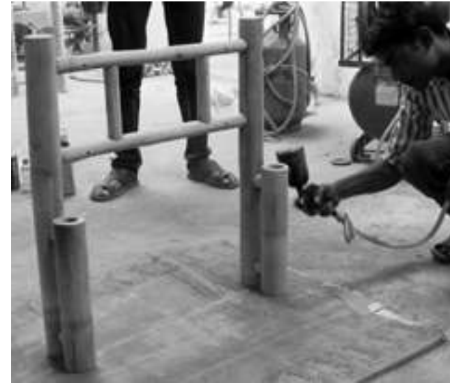
Step 8: Finish the structure by using mellamine.
