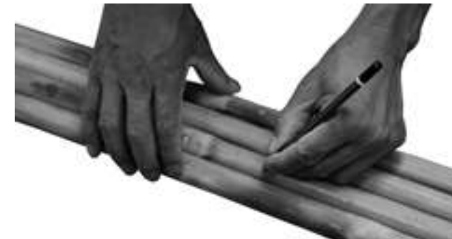
Step 9: Similarly mark on all the bamboos
