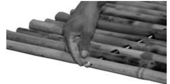
Step 22: Lock with a nut on the other end.
