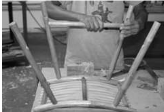
Step 23: Fix the tie member between the legs.
