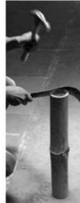
Step 10: Fix hook through the hole on to the topper bead
