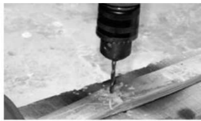
Step 9: Drill into the centre
