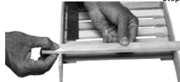
Step 17: This is the handle- fix it with an adhesive.
