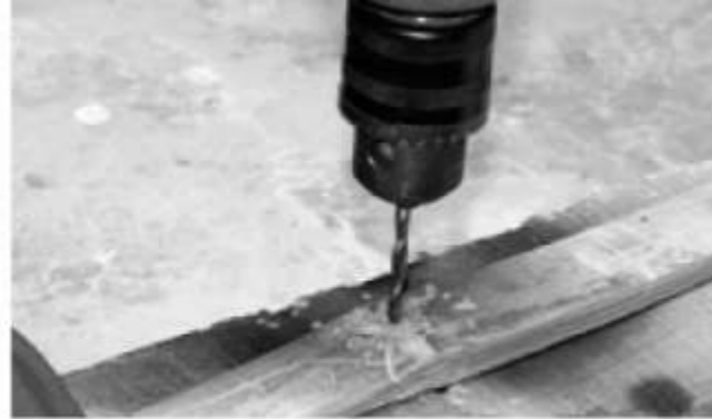
Step 7: Drill hole in the center of top sliver
